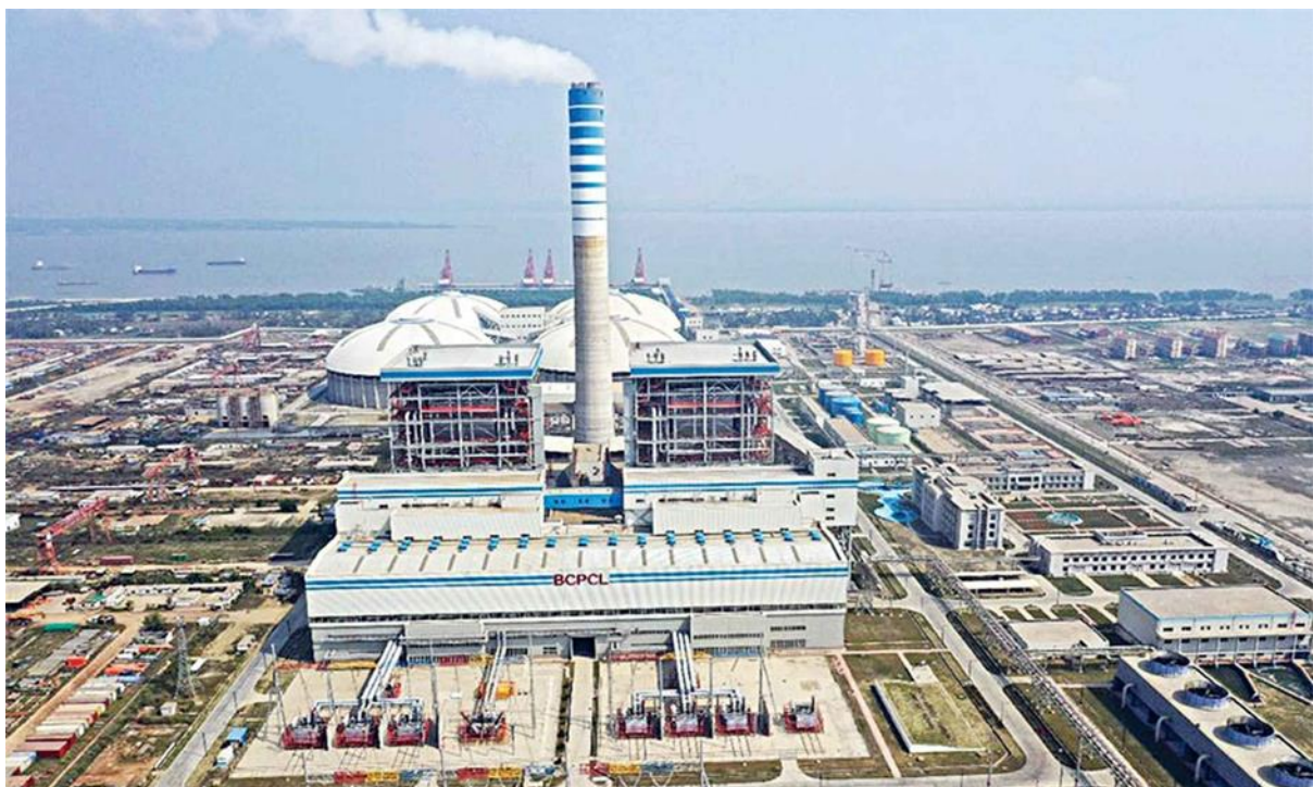
Figure 29-5: A View of the 1320MW Coal-Fired Power Plant in Dhankhali Area
